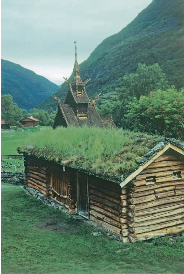
Figure 3.9 Notched log farm building, with turf roof. A stave church is beyond. Borgund, Norway.
