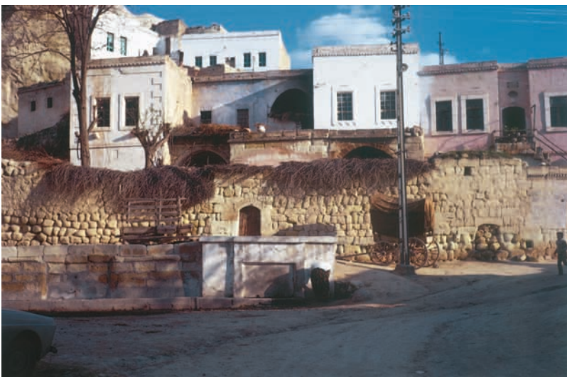
Figure 12.5 Rebuilding of houses below the rockfall. Cavusin, Turkey.
